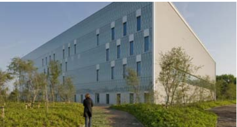
ORGANON PRODUCTION FACILITY, Oss
